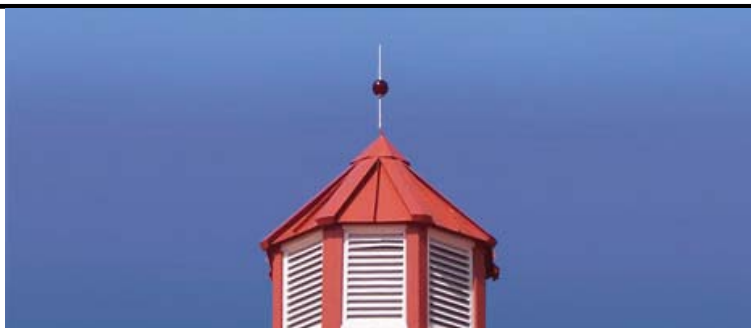
The lightning rod mounted atop this cupola intercepts lightning and protects a building during electrical storms.
