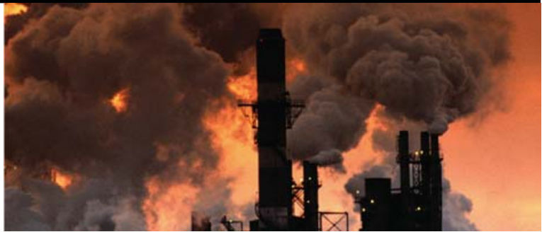
Polluting smokestacks. Electrostatic precipitators could electrically charge this particulate matter and use electric fields to remove it from the effluent.
