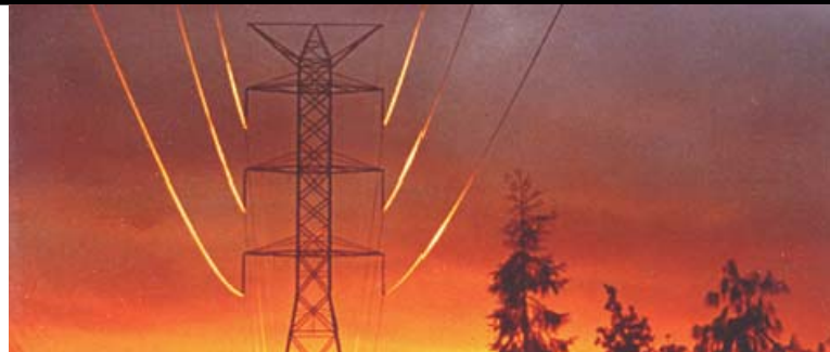
Power transmission lines conduct AC current at high voltages. Transformers convert this current from one voltage to another.
