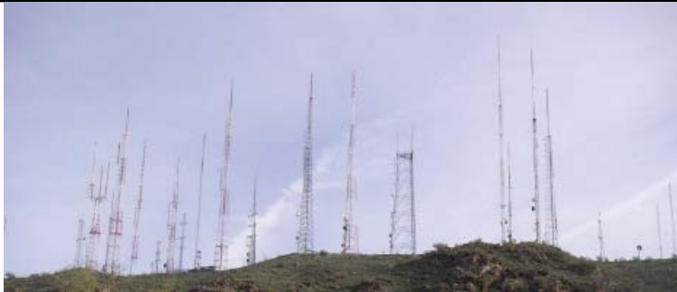
Radio-wave transmitters. A cable carries a modulated electric signal to the dipole antenna rod assembly visible at the top of each tower.
