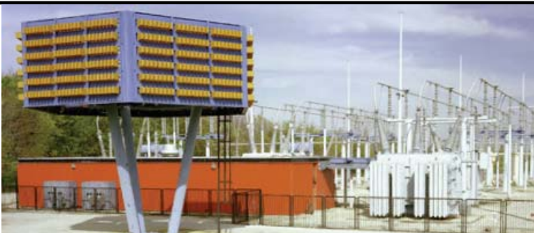
The “capacitor tree” (left) at the Fermilab National Accelerator Laboratory stored huge amounts of energy for high-energy accelerator experiments.
