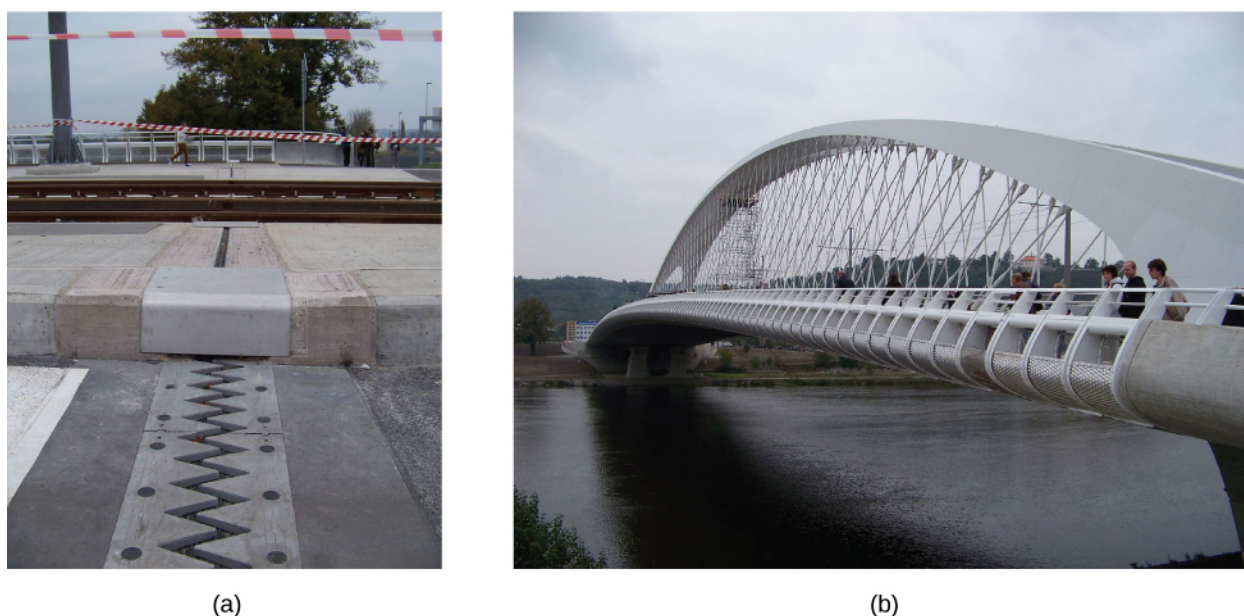
Figure 1.5 (a) Thermal expansion joints like these in the (b) Auckland Harbour Bridge in New Zealand allow bridges to change length without buckling. (credit: modification of works by “ŠJů”/Wikimedia Commons)
